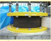
Base isolation system (laminated rubber isolater)
