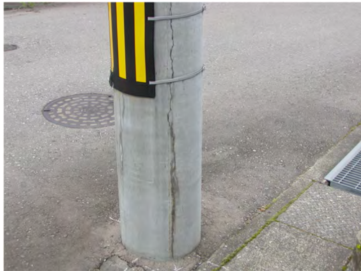
Figure 11. Photograph of an external appearance of vertical cracks.
