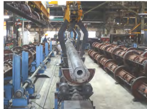
16-4 Formwork removal (upper side)
