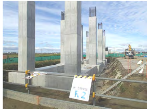
18-4 Photograph of a viaduct in the Hokuriku Shinkansen construction
