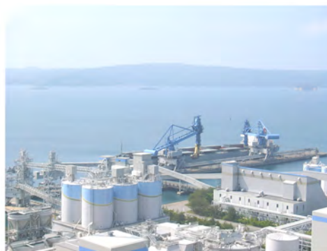
Figure 1. Photograph of an overview of centrifugal machine with fly ash silo.
