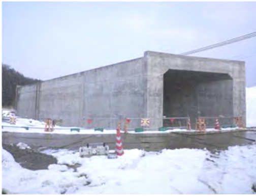
18-1 Photograph of a box culvert in the public works
