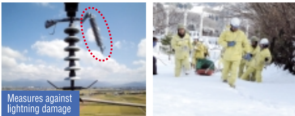
Lightning arrester for transmission
