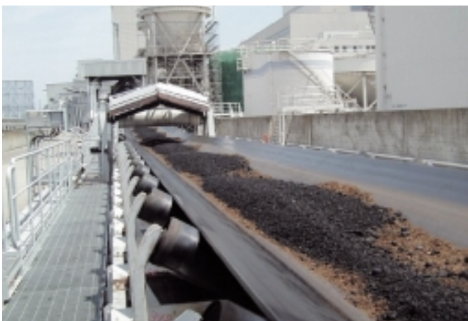
▲Woody biomass fuel being transported (Tsuruga Thermal Power Station)
