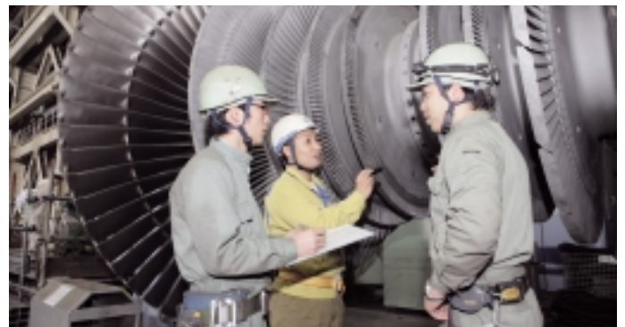
▲ Reliable performance of inspection by making use of "inspection classification tables" (Tsuruga Thermal Power Station)
